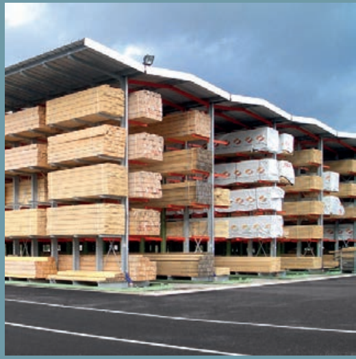
Rack-clad warehouse at a large timber merchant. Roofing from corrugated steel sheeting, with clear panels. Designed as a narrow-aisle warehouse incl. guide rails.
