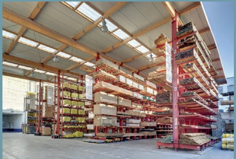
Open rack-clad warehouse. Combination of cantilever and pallet racks as a load-bearing construction for the roof. Bathed in light and with great span for truck passage.
