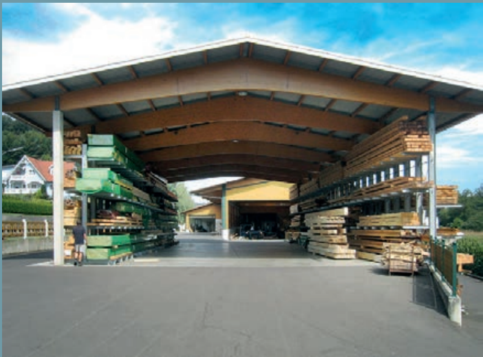
Open cantilever rack-clad warehouse with two double rows of galvanized cantilever racks. With modern saddle roof construction and corrugated sheet metal covering. Large foundation slab.
