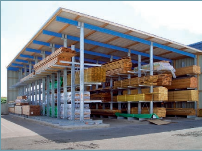
Halfway closed cantilever rack-clad warehouse with hot-dip galvanized racks. Roof and wall of corrugated steel sheeting. Extension to an existing warehouse
