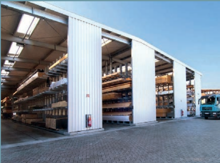
Timber storage with roof and wall panelling. Completely galvanized cantilever racks with guide rail as narrow-aisle warehouse. Clear panels in each aisle.
