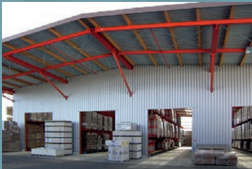
Racking Warehouse Construction - closed design: Including roof covering and wall panelling. The installation of doors, emergency doors and drainage completes the racking warehouse construction.
