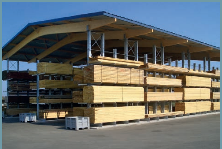
Open cantilever rack-clad warehouse with three double row galvanised cantilever racks. Modern saddle roof construction with 10 m span.
