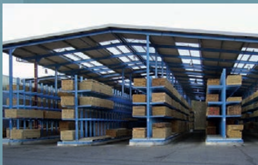
Racking Warehouse Construction - open plan: From conventionally covered rack systems to open rack-clad warehouse. Complete with roof cladding and partial panelling.
