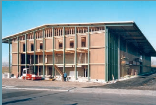
Racking Warehouse Construction - closed design: Including roof covering and wall panelling. The installation of doors, emergency doors and drainage completes the racking warehouse construction.
