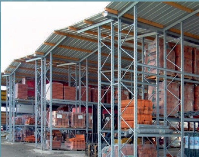
Open pallet rack warehouse for the storage of building materials. Double entry rack, fully galvanised, mounted on block foundations.
