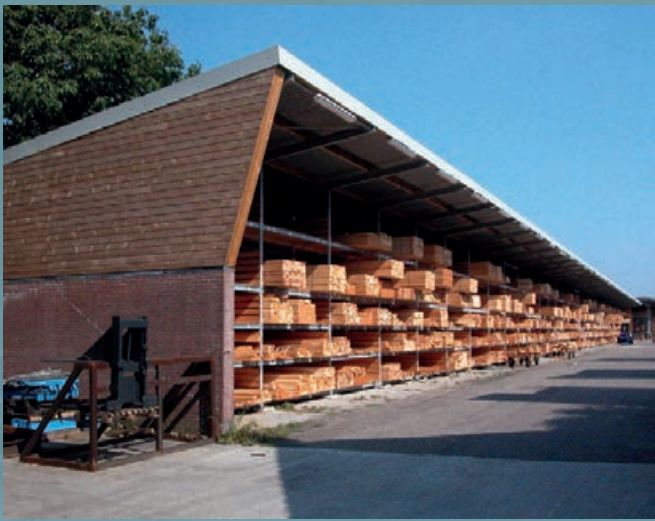
Closed on three sides pallet rack-clad warehouse for the storage of timber with different assortments and dimensions in depth direction. Large roof projection.
