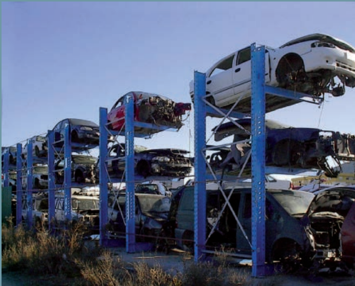
Compact cantilever racks for the storage of end-of-life vehicles in the outdoor area. No rust build-up occurs as with box profiles through the use of steel profiles.
